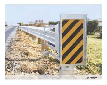
A picture of an ET-Plus end terminal installed on a W-beam guardrail of an unspecified height, taken from the expert report of Dr. Marthinus van Schoor, one of the Turgeons' proposed expert witnesses. See Doc. No. 46-7 at 25.
